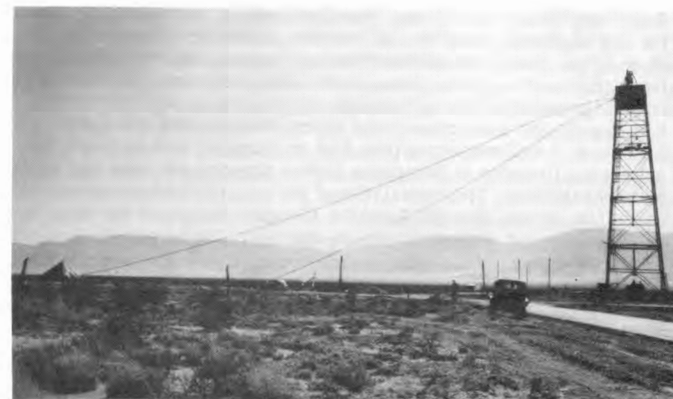
Figure 6. 100-ft tower and coaxial cables (TR-278).
