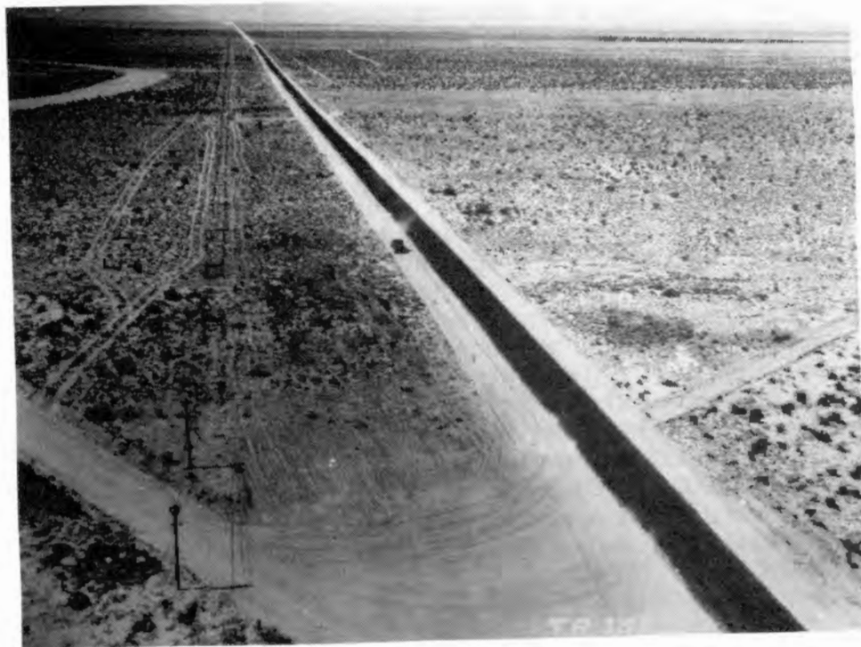
Figure 41. Paved road—South alignment (TR-283).
