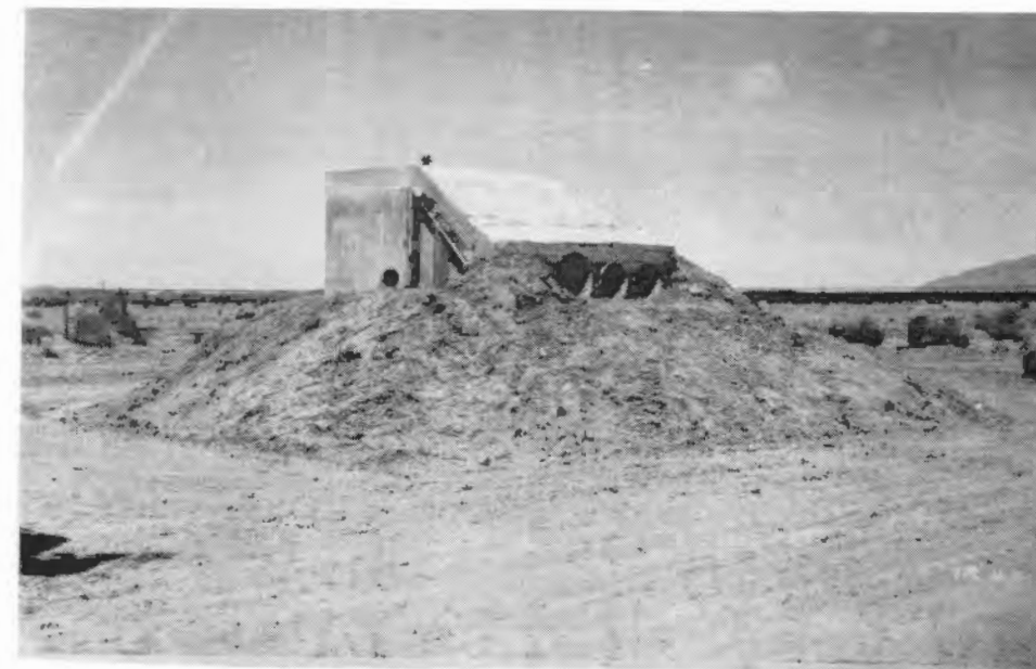
Figure 3. The bunker at North 800 before the test (TR-43).
