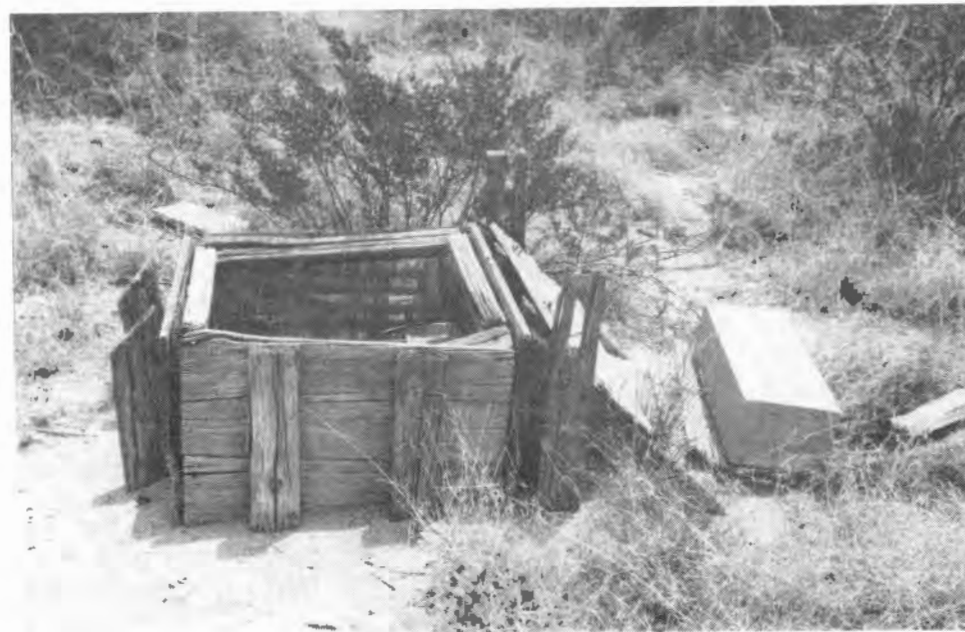
Figure 13. Type B gamma sentinel box, 1997. Note counterweight (photo by Stephen P. Merlan).
