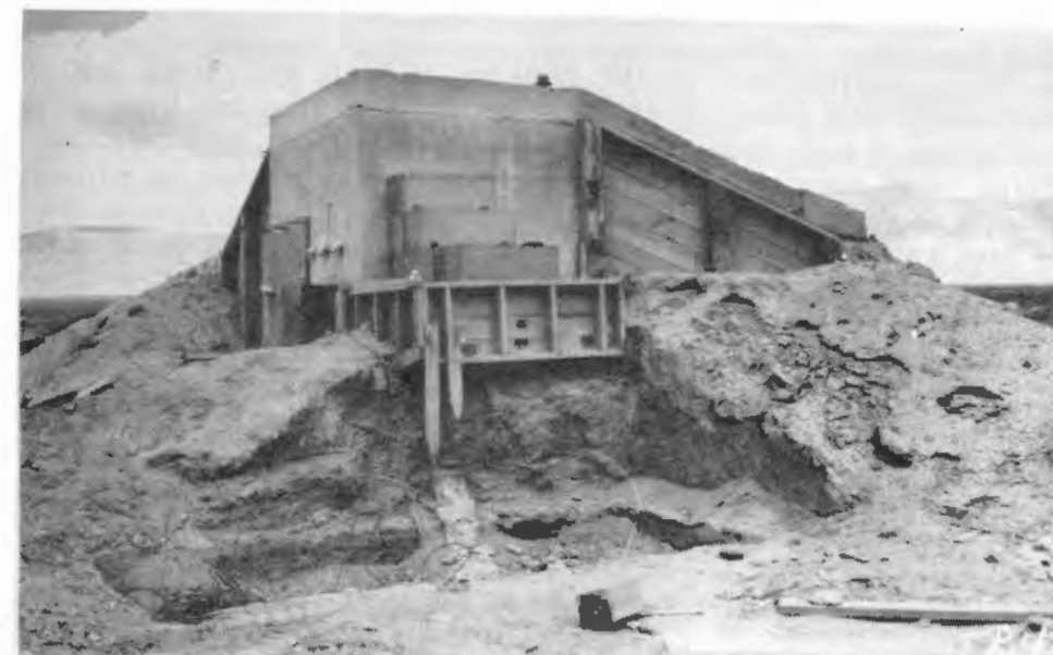
Figure 4. The bunker at North 800 after the test (TR-424).
